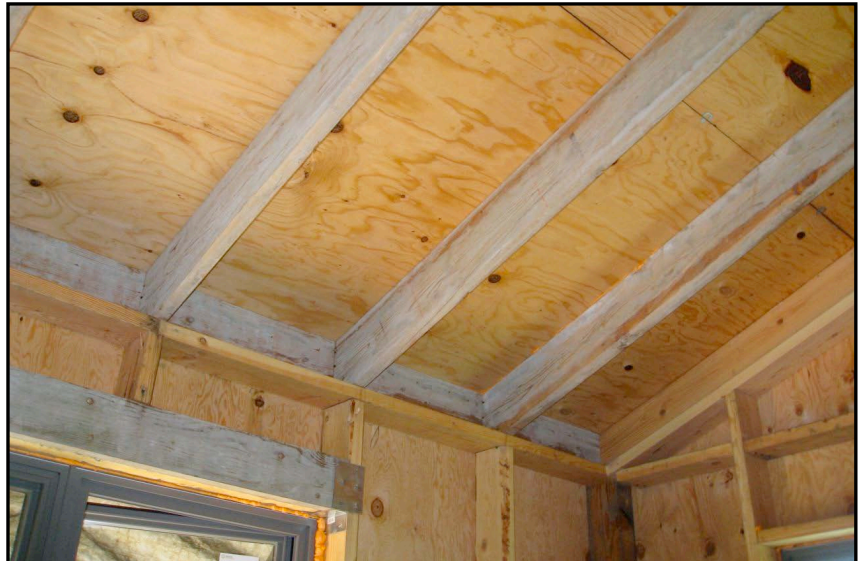
Source: Beyond Efficiency Inc. – CLAM Blue2 House Stacked 24" framing, single top plate, header hangers, no trimmers, no unneeded cripple studs, no header on non-bearing wall
