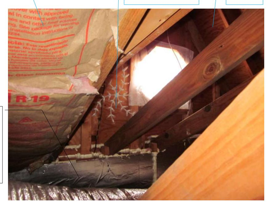
Knee wall that I batt insulated then foam boarded to wall off section of attic over front porch and therefore reduce the size of my 'conditioned attic' project
