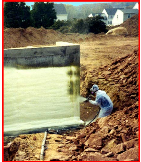
Spray Application to Exterior Foundation Wall
