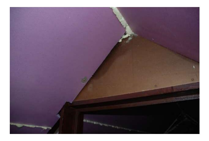
Initially at a handful of spots you would only see this at the very top: There's moisture apparently escaping from behind the foam and condensing on the XPS surface:
