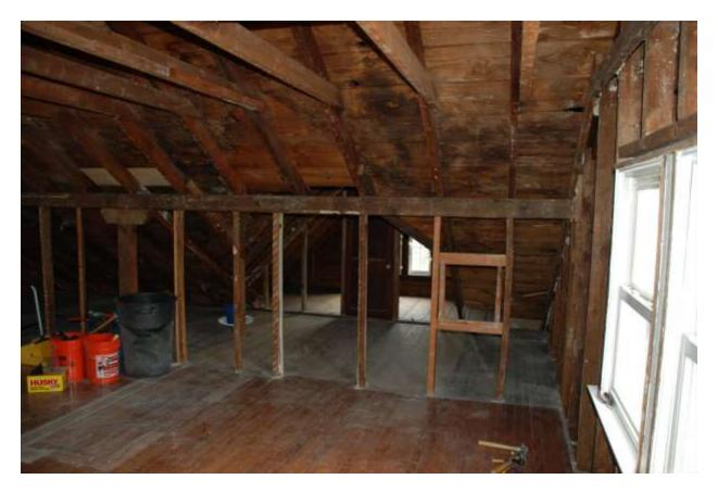
The small windows there are above porch which is not conditioned but has also been gutted and insulated using XPS. There's a chance moisture travels up those walls where the old door is still hanging.
