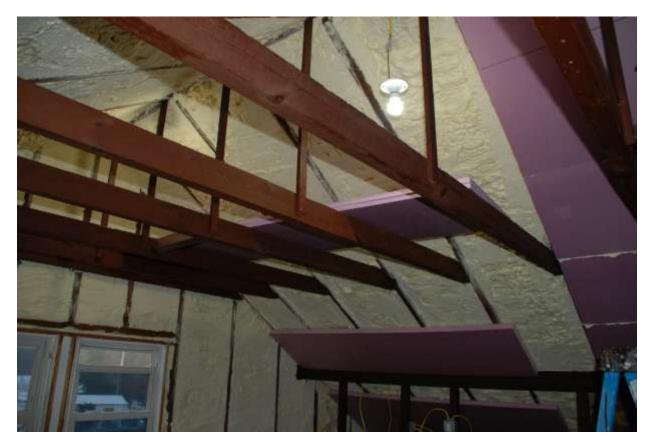
I used 'great stuff' from the can to seal between the XPS boards. The sealing process was quite efficient and quick. Water penetrated only from a handful of places very slowly. Each board at the top had a lot of water behind it and we had no idea... The spray foam was soaked.
