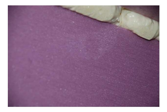
Was the foam not installed correctly? The foam was installed when the RH and hence dew point were relatively high. 70F air temp at weather station, 65F dew point, and over 24h of over 84% RH before spray foam was applied:
