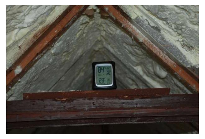
Based on what I have seen the house so far I have reason to believe the moisture is coming out of the foam. It feels that way, too. So I did an old trick and taped thick, transparent plastic on the foam and stuck a thermometer inside. I also had another thermometer (the one above) as control point:
