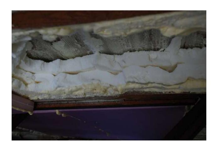
Poor adhesion between layers and large voids in-between:
