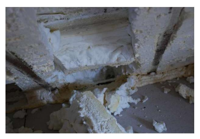
This would also explain the results of my plastic sheet experiment. Plastic was taped airtight over foam in the morning with a thermometer stuck behind the plastic. The RH shot up to 99% within 3-4 hours. The plastic later condensed from the inside (condensation occurred inside the plastic between plastic and foam) 26C = 79F:
