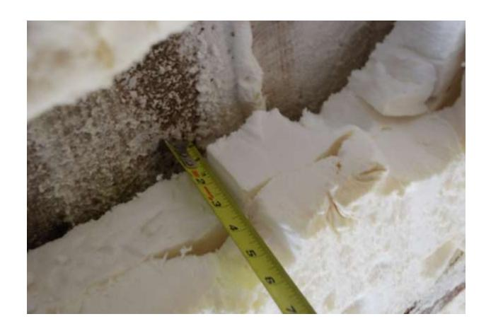
The moisture appeared to be coming from down there, the soffit. After I opened this a few days ago, the RH in the upper floor is fine! I suspect the moist air was coming in behind the foam where it condensated at night. The water and vapors were absorbed by the foam and accumulated over time.
