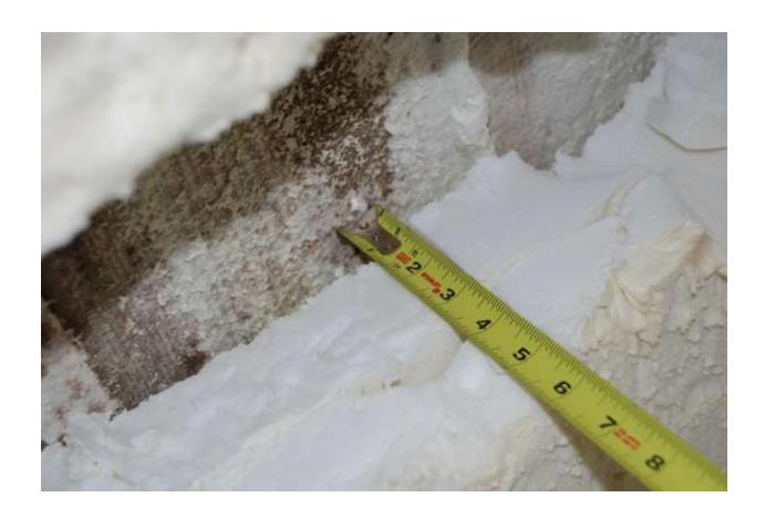
Here we are looking up towards ridge, you can see the gap at top right is even bigger, that's right under the ridge. You can also see voids between the two layers.
