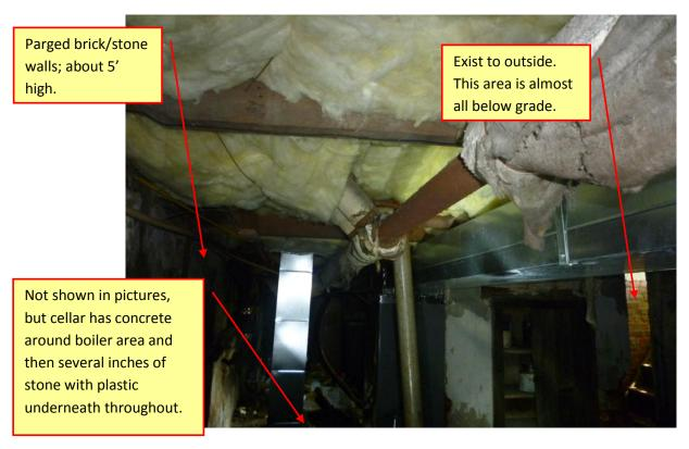
^ "Newer" section – difficult to see, but shows the more structured foundation wall to the left and access stairs to right. Also shows HVAC and chimney foundation (has recessed wood cabinet).
