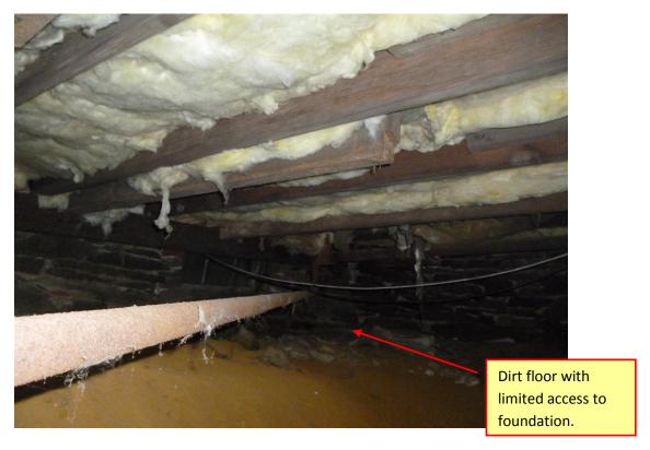
$^{\wedge}$  Original section of the house showing additional low access areas under  $\mathbf{1}^{\text{st}}$  floor and with newer joists.
