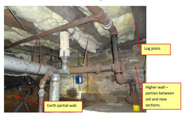
^ Original section of the house showing typical other wall with more vertical structure and also showing old log joists.
