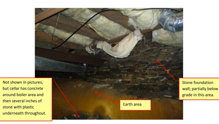
^ Original section of the house showing soil and stacked stone foundation and old log joists.
