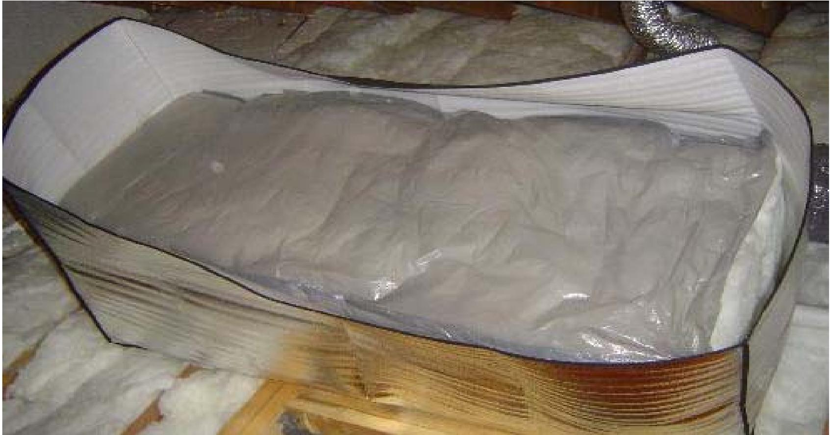
**Insert R-50 fiberglass into reflective shield.**
