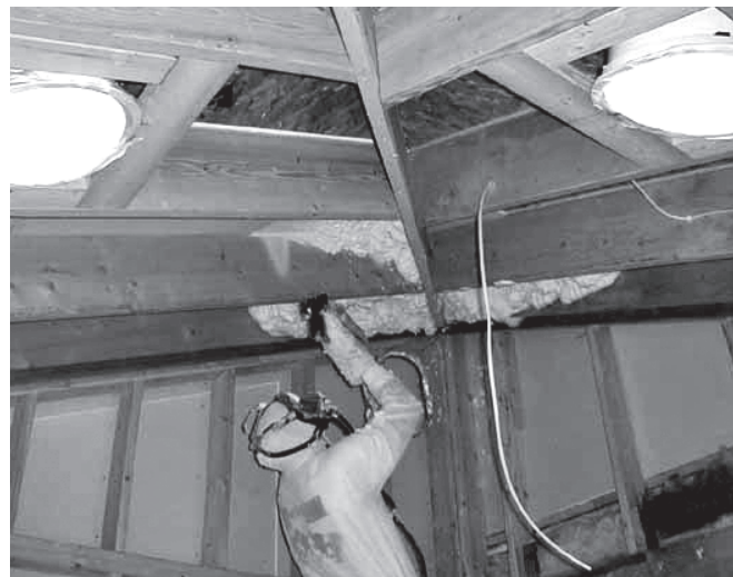
Figure 5. When Icynene is installed in a cold climate, the manufacturer recommends the installation of an interior vapor retarder. [Photo credit: Energy Smart Insulation]
