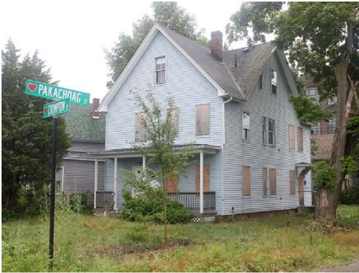
Worcester three-family home before construction
