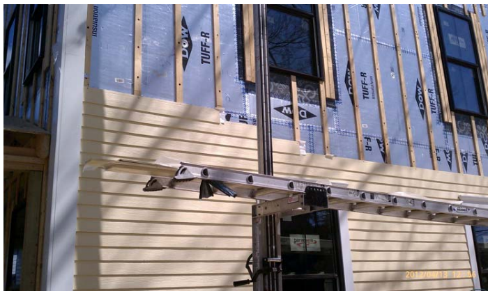
New Siding attached over furring strips
