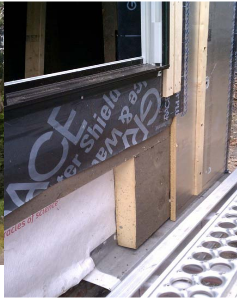
Installing two 2" layers of foil-faced rigid foam insulation (w/ staggered joints)
