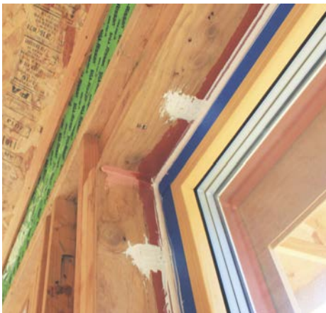
The interior sealant joint (white) is easily inspected from the interior. Special care must be taken to seal around window clips. Blower door testing can help reveal pinhole leaks at this critical seal. Photo courtesy of Skylar Swinford, Hammer & Hand.
