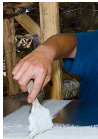
Above: Paint mastic (a thick, gooey substance) onto the duct seams and joints. (Photo source: Habitat for Humanity, Lakeland, FL)
