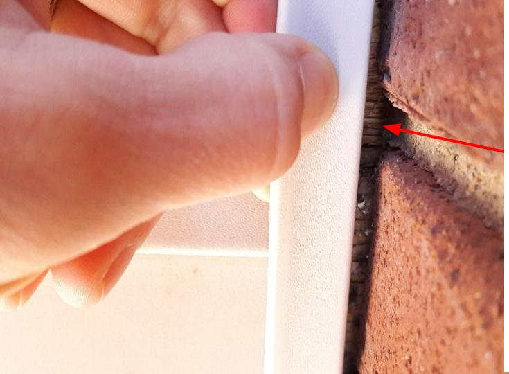
Detail of chimney to wall intersection. Vinyl siding J-channel pulled pack. Exposed is unsealed sheathing to brick connection. Plywood appears sun bleached and not in great shape. The situation in this photo continues at all points of inspection within reach. There is tyvek under siding, but not visible here.
