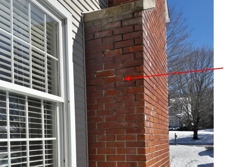
Spalling at face of bricks. Chimney top and flue liner was repointed with concrete and aluminum rain cap two years ago. Spalling continues. -My understanding is I have water intrusion somewhere still. Or is it flue gasses condensing? Furnace is oil fired 126K BTU Peerless boiler with a Beckett AFG burner.
