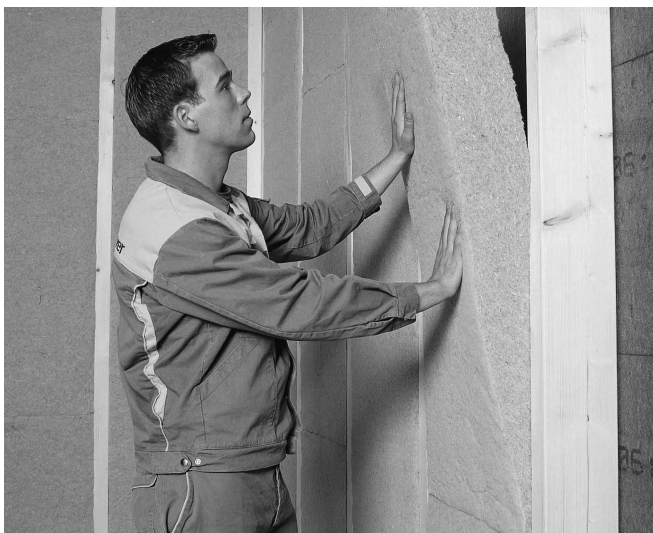
Figure 4 — Hemp fiber batts, like these Florapan batts from Isover, are stiffer than fiberglass batts. Hemp insulation is non-irritating, and can be installed without gloves or a facemask.
