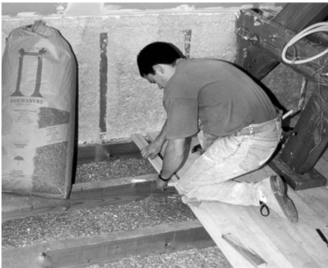
Figure 3 — Loose-fill insulation made from hemp hurds, like the Isochanvre Isolation in this photo, can be poured straight from the bag into wall cavities or joist bays.
