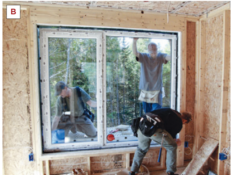
Figure 5. The window bucks were protected with flashing tape (A) before the window units were installed (B). Windows were secured with metal clips (C) and frames were taped and air-sealed (D).
