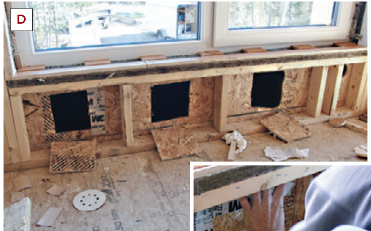
Figure 8. Where possible, wall cellulose was blown into the I-joint cavities from the attic (A), through holes cut in the OSB air barrier (B). Where windows interrupted the cavities, the insulation was blown from below (C). After the insulation was installed, the crew re-installed the cutouts and sealed the holes (D, E). Later, Roxul mineral wool batts were installed in the inner 2x4 wall, increasing overall wall R-value to 58.7.
