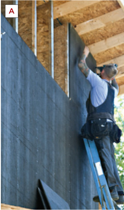
Figure 4. A secondary asphalt-faced fiberboard sheathing (A) was installed over the wood I-joists to retain the cellulose insulation. Edge gaps were sealed with spray foam (B), then the shell was covered with housewrap (C).
