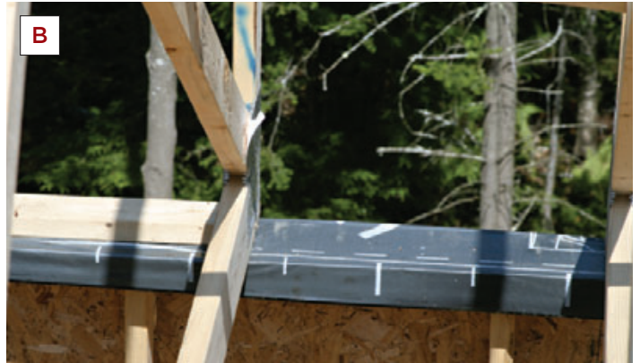
Figure 1. Before setting the mono-pitched roof trusses (A), the carpenters attached an OSB gusset to the top plate of the 2x4 bearing walls (B); peel-and-stick flashing seals the outside top corner of the wall. The roof was conventionally framed (C) and covered with asphalt shingles.
