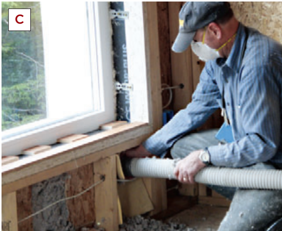
Figure 8. Where possible, wall cellulose was blown into the I-joint cavities from the attic (A), through holes cut in the OSB air barrier (B). Where windows interrupted the cavities, the insulation was blown from below (C). After the insulation was installed, the crew re-installed the cutouts and sealed the holes (D, E). Later, Roxul mineral wool batts were installed in the inner 2x4 wall, increasing overall wall R-value to 58.7.
