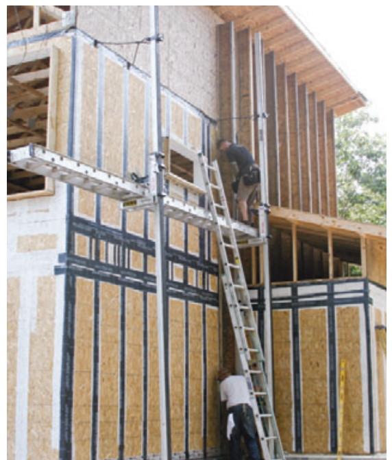
Figure 2. The author applied strips of Vycor membrane at stud locations (above) to ensure that the fasteners securing the vertical I-joists (right) would not create leaks in the OSB air barrier.
