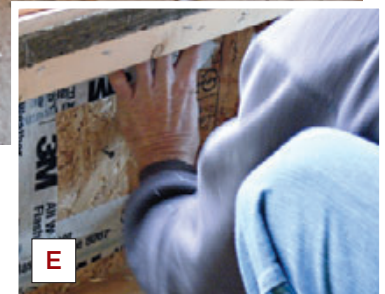
Figure 8. Where possible, wall cellulose was blown into the I-joint cavities from the attic (A), through holes cut in the OSB air barrier (B). Where windows interrupted the cavities, the insulation was blown from below (C). After the insulation was installed, the crew re-installed the cutouts and sealed the holes (D, E). Later, Roxul mineral wool batts were installed in the inner 2x4 wall, increasing overall wall R-value to 58.7.
