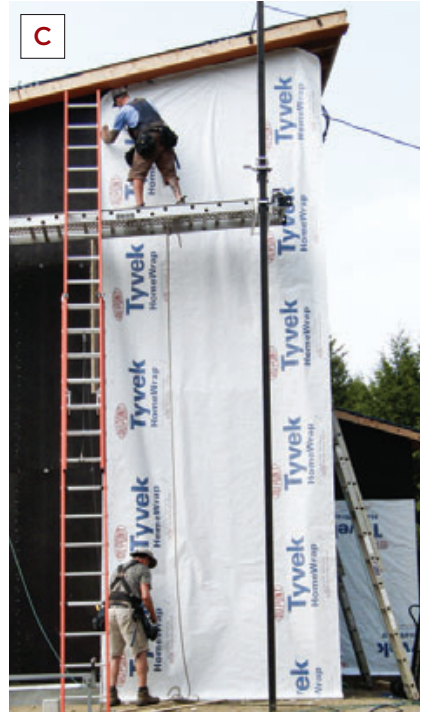
Figure 4. A secondary asphalt-faced fiberboard sheathing (A) was installed over the wood I-joists to retain the cellulose insulation. Edge gaps were sealed with spray foam (B), then the shell was covered with housewrap (C).
