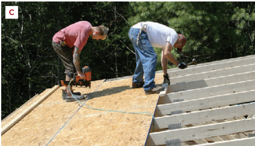
Figure 1. Before setting the mono-pitched roof trusses (A), the carpenters attached an OSB gusset to the top plate of the 2x4 bearing walls (B); peel-and-stick flashing seals the outside top corner of the wall. The roof was conventionally framed (C) and covered with asphalt shingles.
