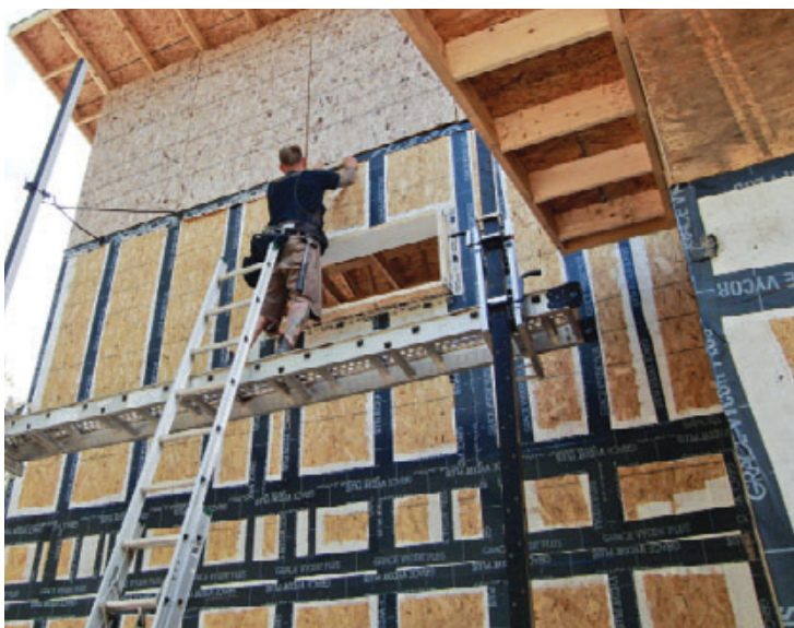
Figure 2. The author applied strips of Vycor membrane at stud locations (above) to ensure that the fasteners securing the vertical I-joists (right) would not create leaks in the OSB air barrier.
