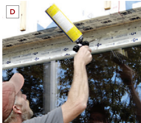
Figure 5. The window bucks were protected with flashing tape (A) before the window units were installed (B). Windows were secured with metal clips (C) and frames were taped and air-sealed (D).
