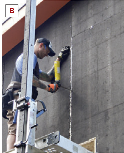
Figure 4. A secondary asphalt-faced fiberboard sheathing (A) was installed over the wood I-joists to retain the cellulose insulation. Edge gaps were sealed with spray foam (B), then the shell was covered with housewrap (C).
