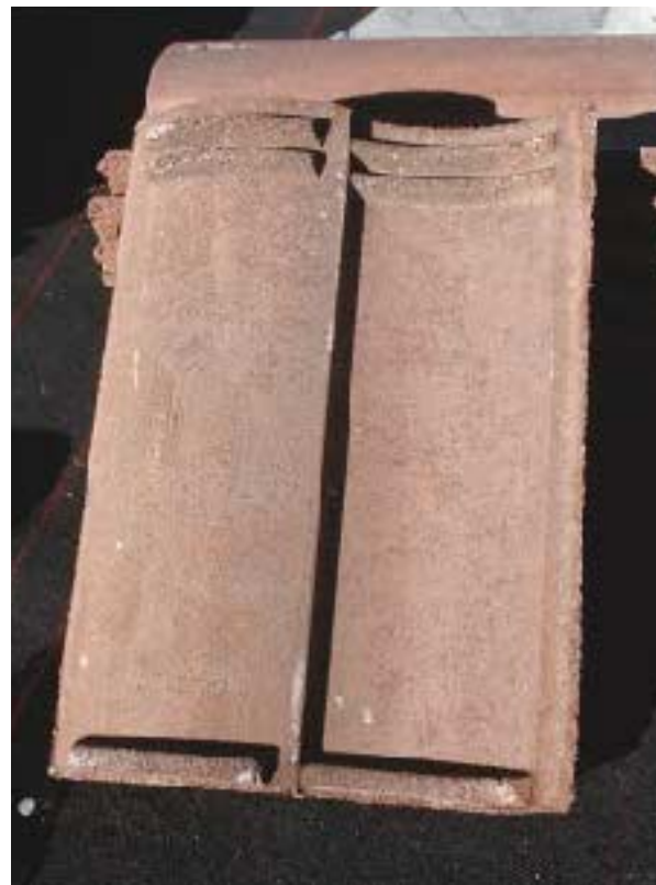
Figure 4. Birdstop metal is the flashing that raises the heel of the first course of tiles while closing the openings below it (left). The underside of an S-tile has two ridges designed to conform to the birdstop metal (right).
