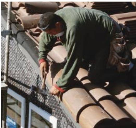
Figure 9. Rakes are trimmed with barrel tiles. Each tile is secured with two nails, which are driven horizontally into the rake board.
