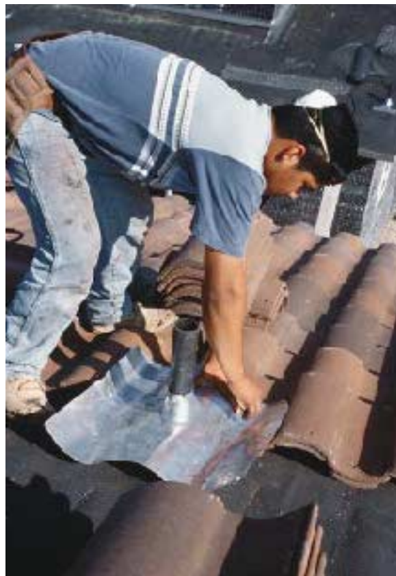
Figure 1. Each plumbing vent receives two layers of metal flashing. The primary flashing is galvanized and is installed at the same time as the asphalt felt (above). The secondary flashing is installed later, when the tiles go on. An S-tile roof gets secondary flashings made of aluminum, which is flexible enough to conform to the curve of the tiles (right).
