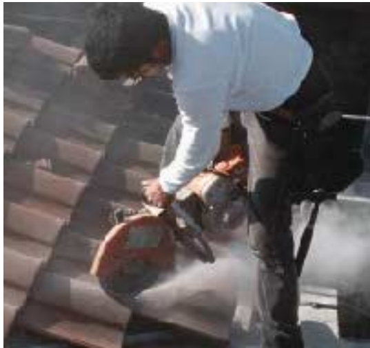
Figure 8. Where tiles intersect a valley, they are cut roughly, so they run a little long. Then a chalk line is snapped, and the tiles are trimmed with a saw.
