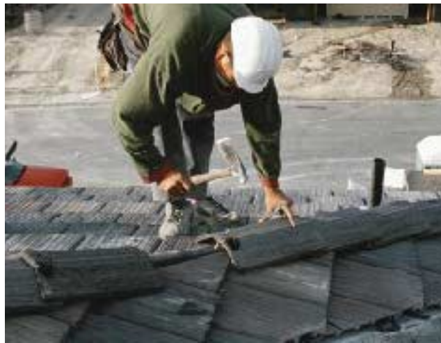
Figure 10. This style of ridge tile is used to trim roofs with flat tiles. Each ridge tile is secured at one end with a single nail and at the other end with asphalt cement.
