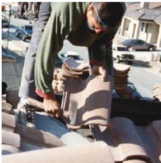
Figure 6. A small corner of tile can often be knocked off with a hatchet (above). Larger cuts are made with a saw equipped with a diamond blade (right).
