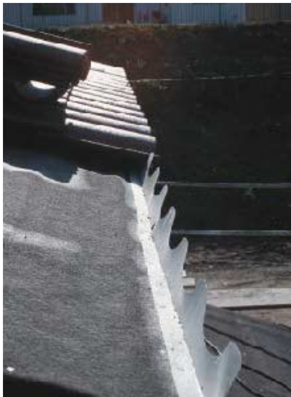
Figure 4. Birdstop metal is the flashing that raises the heel of the first course of tiles while closing the openings below it (left). The underside of an S-tile has two ridges designed to conform to the birdstop metal (right).
