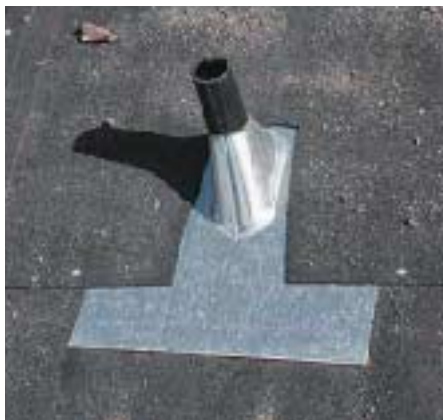
Figure 1. Each plumbing vent receives two layers of metal flashing. The primary flashing is galvanized and is installed at the same time as the asphalt felt (above). The secondary flashing is installed later, when the tiles go on. An S-tile roof gets secondary flashings made of aluminum, which is flexible enough to conform to the curve of the tiles (right).
