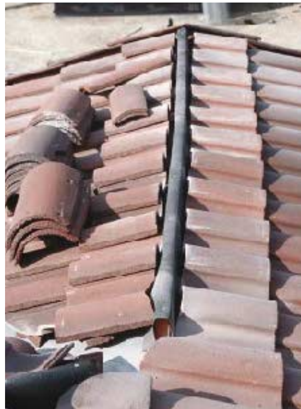
Figure 2. Typically, hip boards — nailers that support the hip shingles — are 2x4s or 2x6s (above). Hip and ridge boards are installed after the roof has been felted and are later separately wrapped with felt (right).
