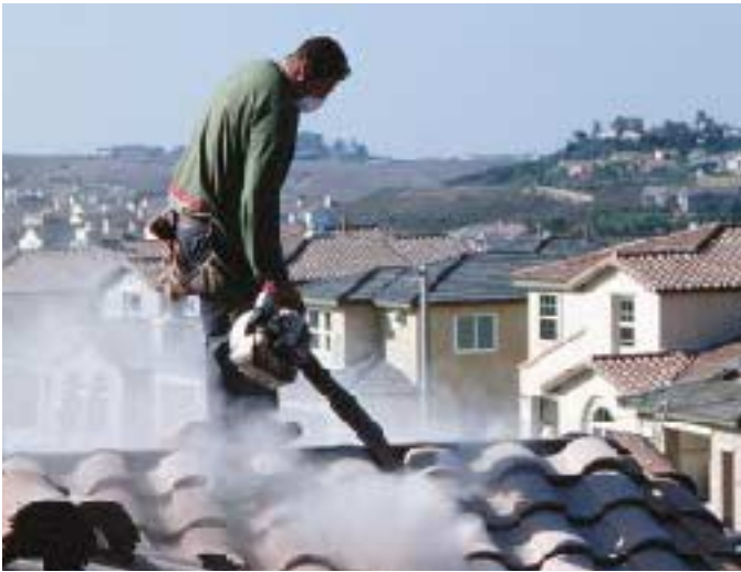
Figure 7. Cutting tiles on the roof leaves fine cement dust, which should be thoroughly removed with a leaf blower. If the dust is left on the roof, it can turn into an unsightly cement paste when it rains.
