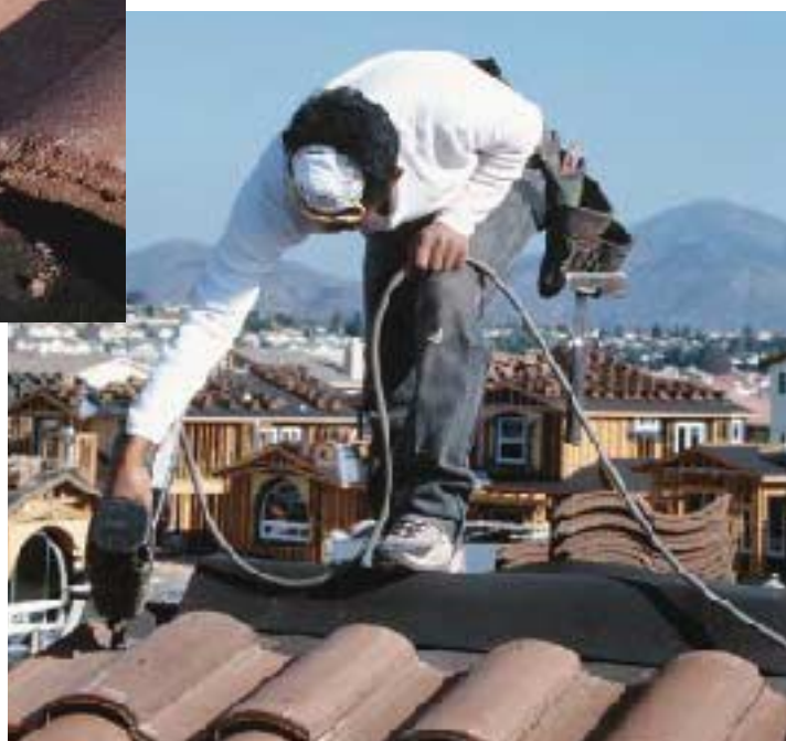
Figure 5. Each S-tile receives a single nail in the lower nail hole (inset above). The upper nail hole is used to secure a cut tile that can't be nailed in the preferred hole. The most efficient way to install tiles is with a nail gun (above).
