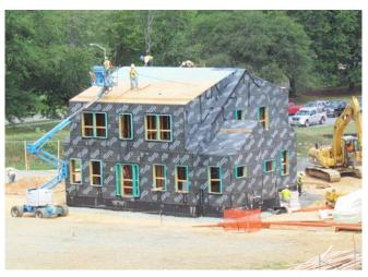
Photograph 1: Ultra Tight House – Advanced frame house sealed with a fully adhered exterior air control layer installed over structural sheathing yields an enclosure with a leakage rate less than 0.5 ach@50 Pa as tested under pressurization or depressurization.
