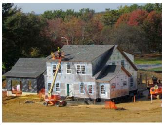
Photograph 2: More Ultra Tight House – Continuous exterior insulation installed over fully adhered exterior air control layer to control condensation at the exterior air control layer – structural sheathing interface. Note that the garage is not attached to the house. Good idea, but typically not possible.
