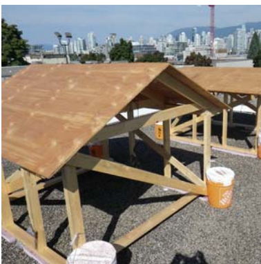
Figure 6: Roof huts under construction with plywood sheathing installed.
