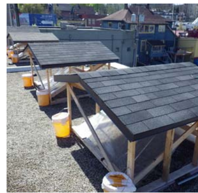
Figure 8: Completed roof huts in place on low-slope commercial rooftop in Vancouver, BC.
