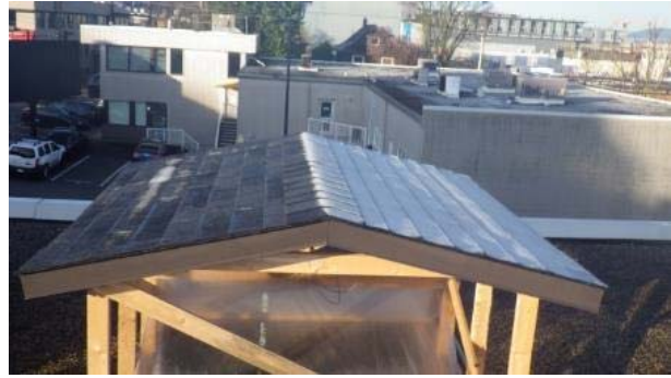
Figure 16: Frost on exterior of shingles and impact of rising sun during morning of January 2, 2013
