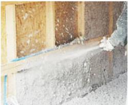
Figure 5: Illustration of cellulose insulation flocking (NrGaïa website, 2013)
