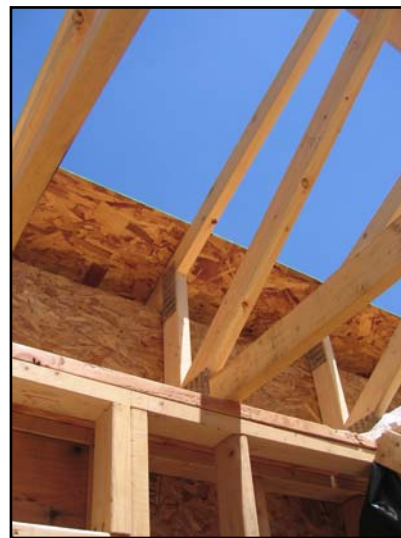
Fig. 4: Raised heel trusses
