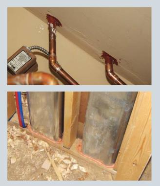
The red caulk around these pipes (top) is approved for use in fire-rated assemblies. The orange polyurethane spray foam around the ducts (above) is not intended for use in fire-rated assemblies, and may or may not be accepted by building officials for sealing penetrations through fire blocking.
