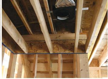
height studs running from the floor deck to the sloped top plate. Under an earlier state code, we had to install fire blocking every 10 vertical feet in these tall bays. That rule has been dropped, but we still have to block where a flat ceiling or attic floor meets the rake wall. With cathedral ceilings, the double top plates serve as fire blocking.
