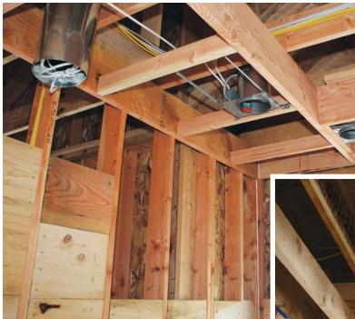
**Figure 1.** The author uses a single 2x10 fire block nailed to the face of the studs for this kitchen soffit — much faster than installing individual blocks in the stud bays (above). Scraps of OSB rim board isolate a dropped ceiling (right) from the stud cavities on its left and the stair stringers beyond. ning a band of sheathing or drywall around the perimeter before hanging the ceiling joists is more efficient than installing individual blocks in the stud bays.
