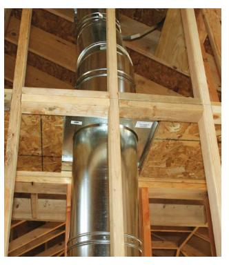
**Figure 3.** To separate the chimney chase from the attic, the author installs a <sup>3</sup>/4-inch OSB fire block at the level of the ceiling. A metal fire stop fills the gap that is required between flue and OSB.
