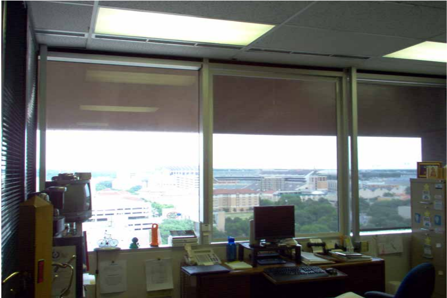
Texas Conservation Commission Building – AUSTIN, TEXAS Left Window – No Inflector Radiant Barrier Window Insulator
