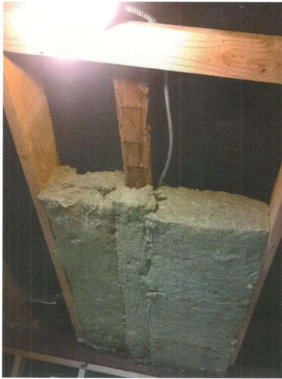
FIGURE 4: ROCKWOOL BATTS PRESS FIT BETWEEN NEW RAFTERS.
