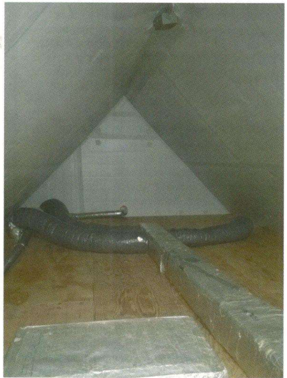
FIGURE 5: COMPLETED ATTIC WITH POLYISO.
