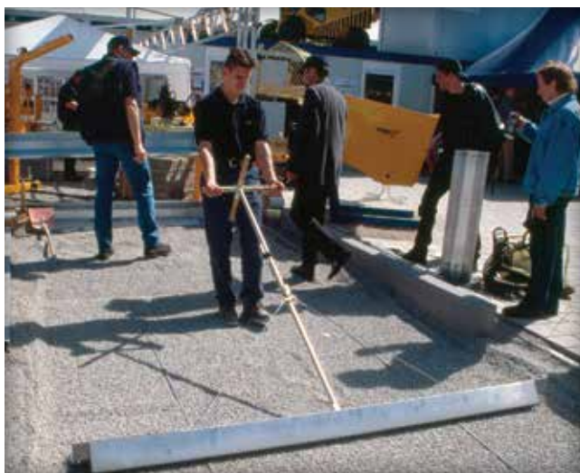
Figure 24. Manually screeding the No. 8 stone setting bed.
