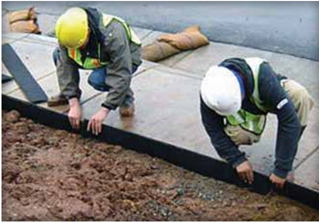
Figure 10. This temporary permeable edging around bare soil replaces silt fencing because it restrains sediment while allowing water to pass.
