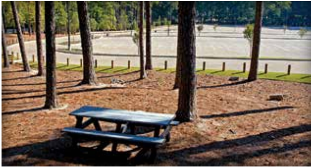
Figure 3. A large PICP parking lot manages an overall site slope of 12% using terraced areas.
