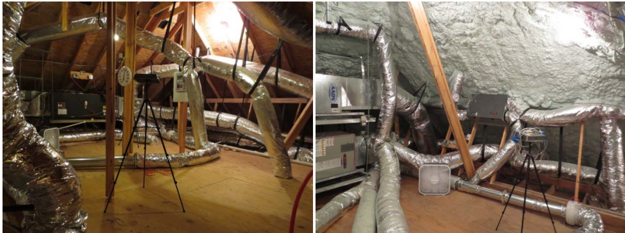
Figure 6. House 1 vented attic (left) and House 2 unvented attic (right)
