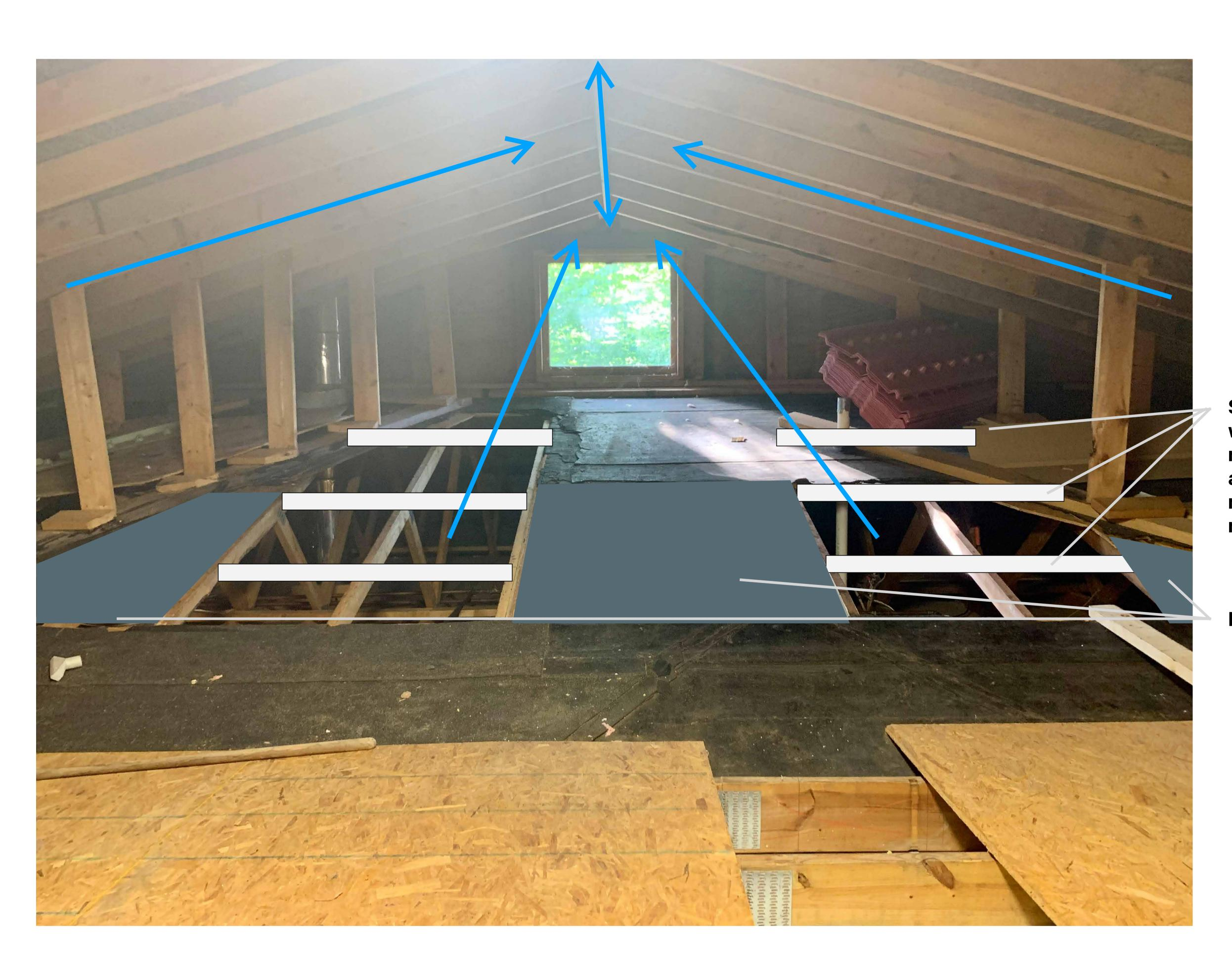
Strap sheathing with 2X4s, to reinforce truss, also allow for air movement up to ridge vent
