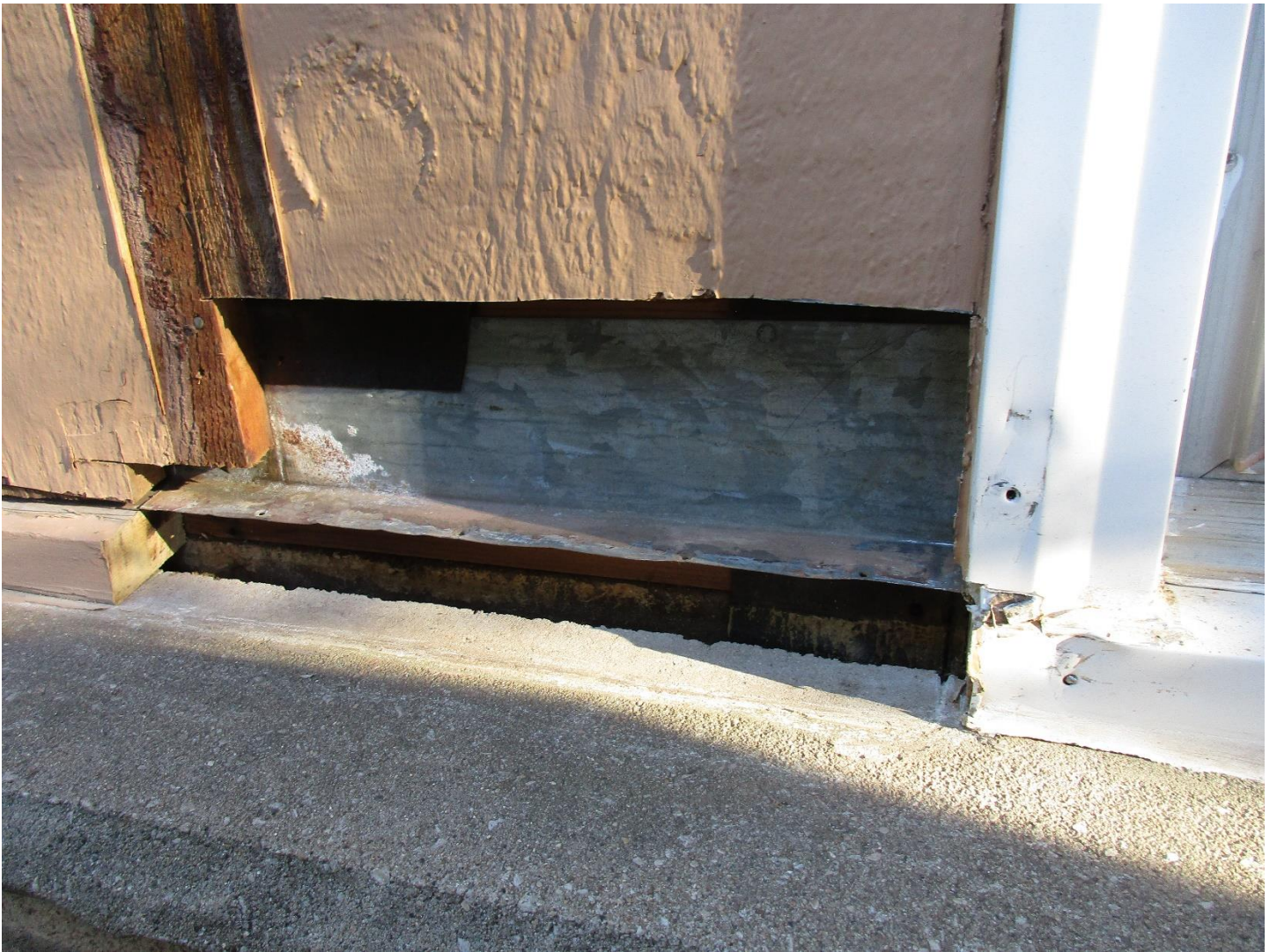
The white aluminum on the right is a window that will be eliminated as part of the project.
