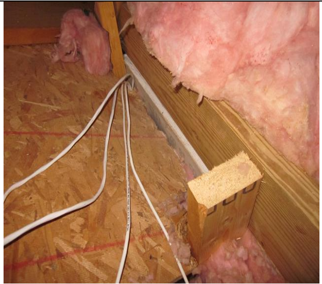
Figure 30-Open wall cavity in attic.
