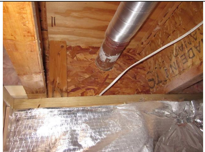
Figure 14-Utility opening in rim band joist.
