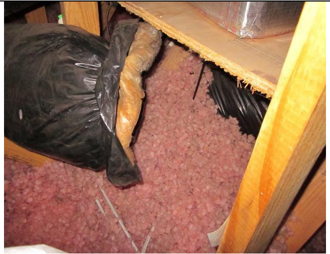
Figure 4-Another line disconnected!
