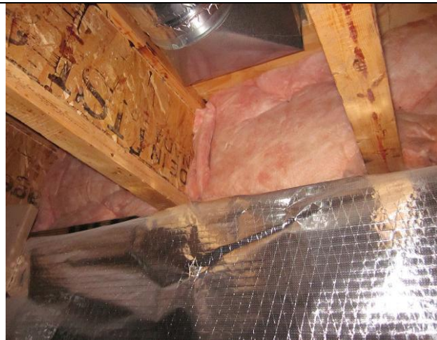
Figure 13-Insulated rim band joist.
