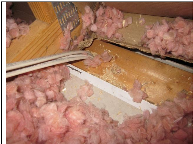
Figure 27-Top plate with electrical holes.
