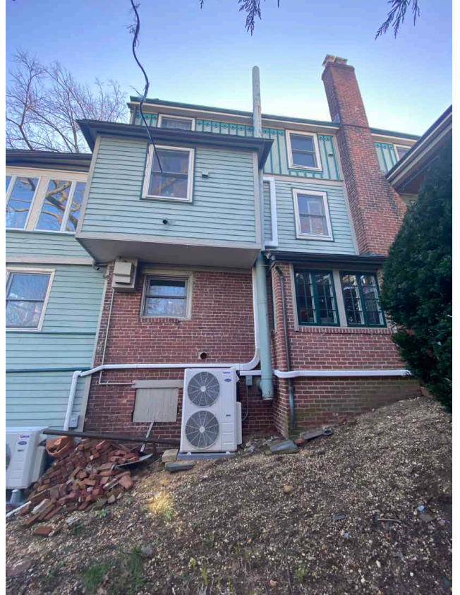
SIDE FACADE (WEST) : VIEW FROM WEST YARD
