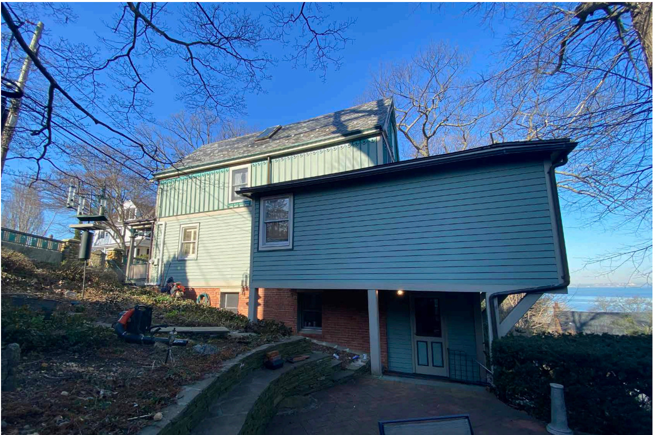
SIDE FACADE (EAST) : VIEW FROM EAST YARD
