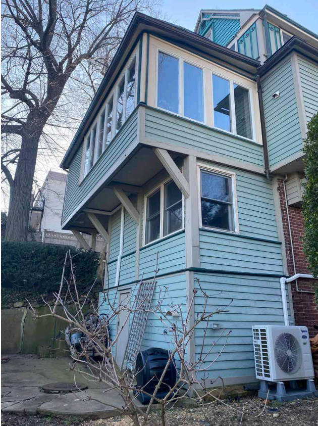
SIDE & REAR FACADE (WEST & NORTH)
