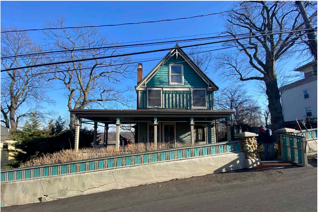
FRONT FACADE (SOUTH) : STREET VIEW FROM 8TH AVE
