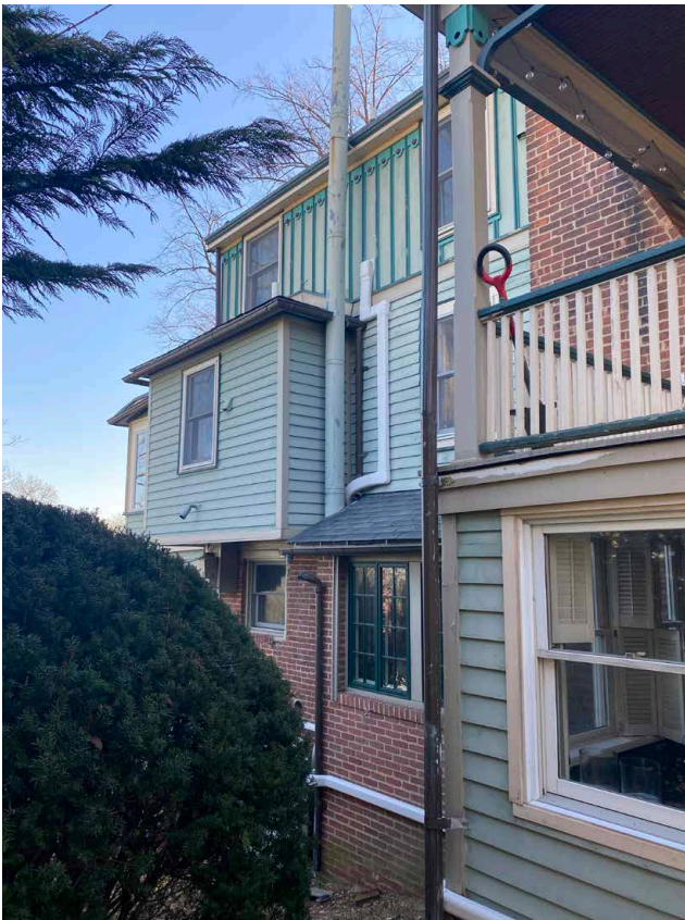
SIDE FACADE (WEST) : VIEW FROM WEST YARD
