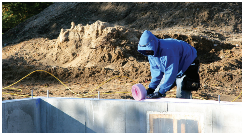
After the foundation concrete cures, sill seal is usually the first thing to be installed. This foam material air-seals the joint between the foundation and the mudsills. In most cases, those mudsills are made of treated lumber.
