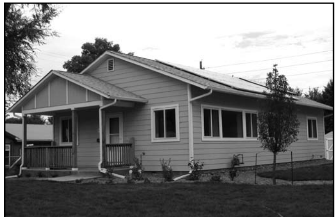
Figure 1. To make them inconspicuous, the photovoltaic modules and solar thermal collectors at the near-zero-energy house in Wheat Ridge, Colorado, were mounted with minimal clearance to the roofing.
