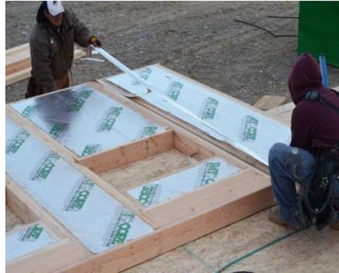
**Step 8. Standing the Walls:** Sheathing can be attached either before or after the wall has been raised, depending on the framer's preference. This flexibility allows framers to choose the sequencing that works best for their specific
