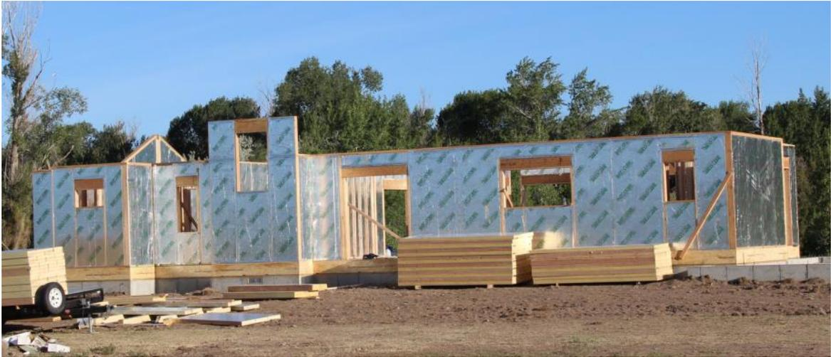
RAYCORE Structural Insulated Wall Panels® are not intended to serve as a finished and exposed surface. Internal surfaces of panels must be covered with a minimum 15-minute thermal barrier, such as 1/2 inch (12.7mm) gypsum wallboard or other approved materials. External surfaces of the panels should be finished promptly with materials that offer protection from sunlight, weather, moisture and all other elements. This ensures the longevity and performance of the wall system.
