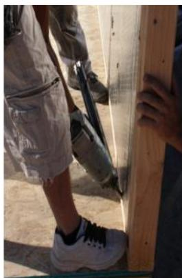
Construction process and project requirements. Apply a continuous bead of foam-friendly construction adhesive to the bottom plate to create an airtight seal between the subfloor and the wall. Securely face nail the bottom plate on both sides to the rim board and floor joists using appropriate fasteners per conventional framing practices and building code requirements.
