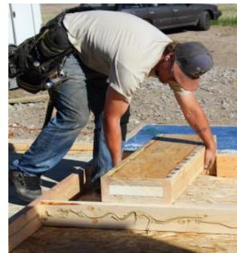
**Step 2. Wall Layout:** Begin by establishing your layout, starting with the corners (see Step 3 & 4). Place lumber, measure, and mark the top and bottom plates. Lay out panels, door and window frames, etc., according to your design plan. This step ensures accurate positioning and alignment of structural components before assembly.
