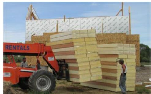
Upon receipt, store the panels in a protected, elevated area and on stickers to avoid ground contact. Use covers or tarps to shield from sunlight, moisture, and the elements. Improper storage could lead to damage, decomposition and possible tolerance issues.
