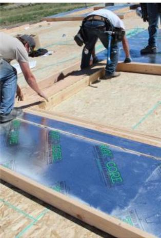
condensation and moisture transfer, maximizing the energy efficiency of the envelope. Fill voids above and below windows with pieces of surplus cut panels to complete the installation.
